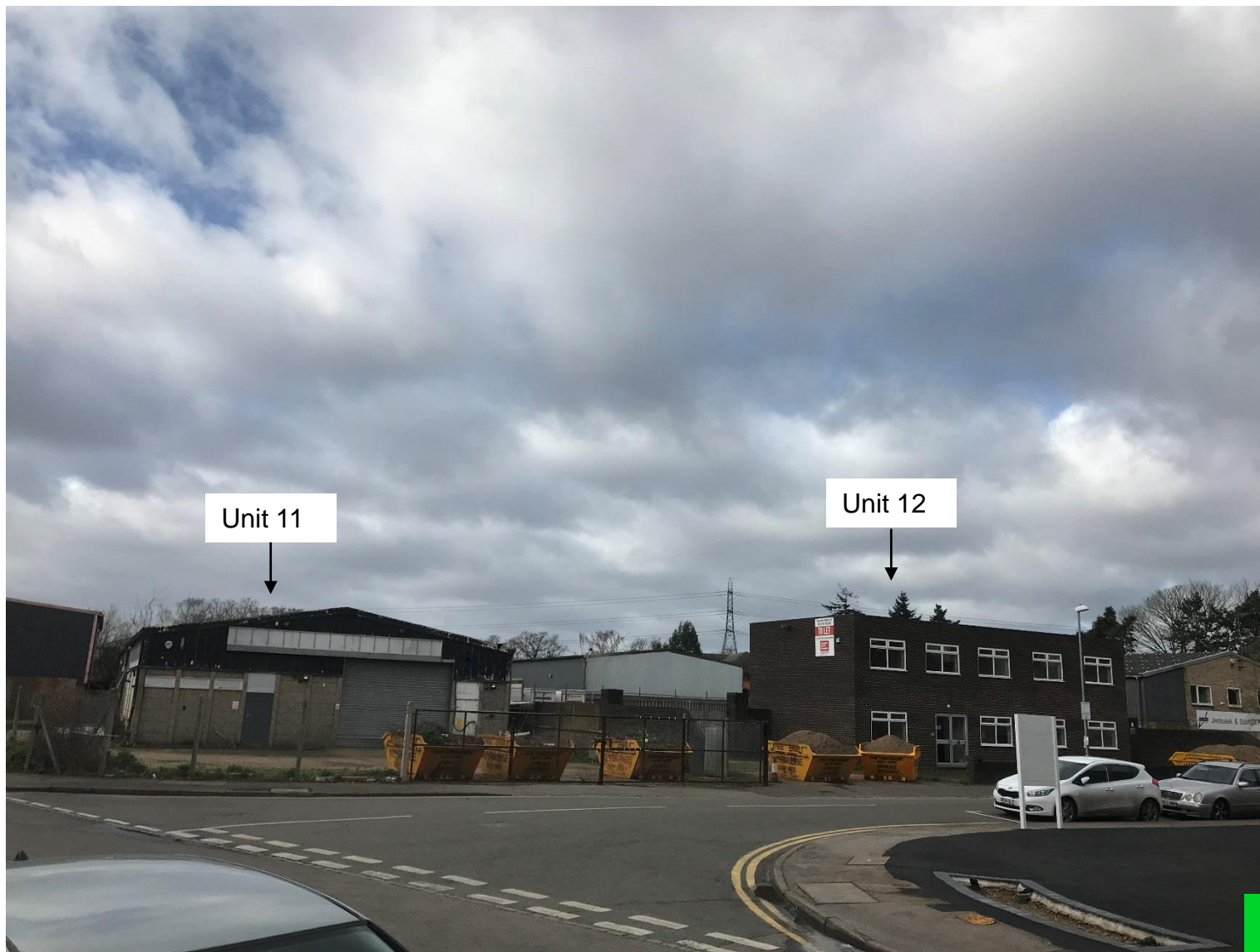
Photo 1: View of Units 11 and 12 looking north-west.
