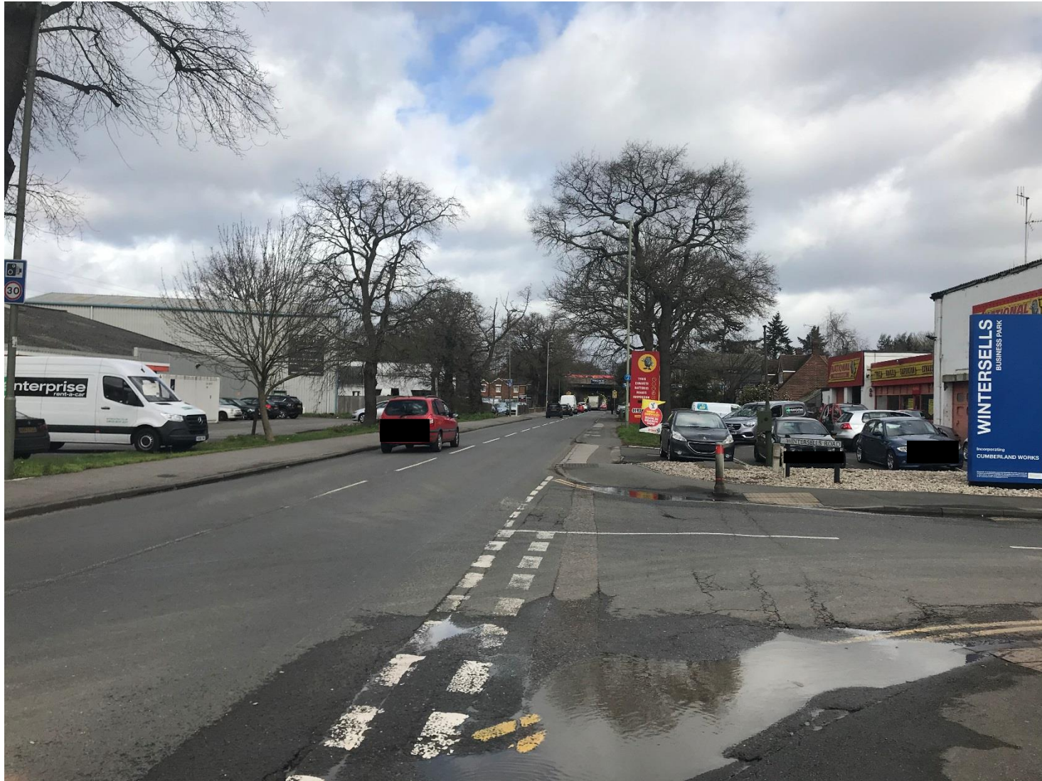
Photo 17: View of the junction of the Wintersells Business Park with the A318 Oyster Lane, looking north.
