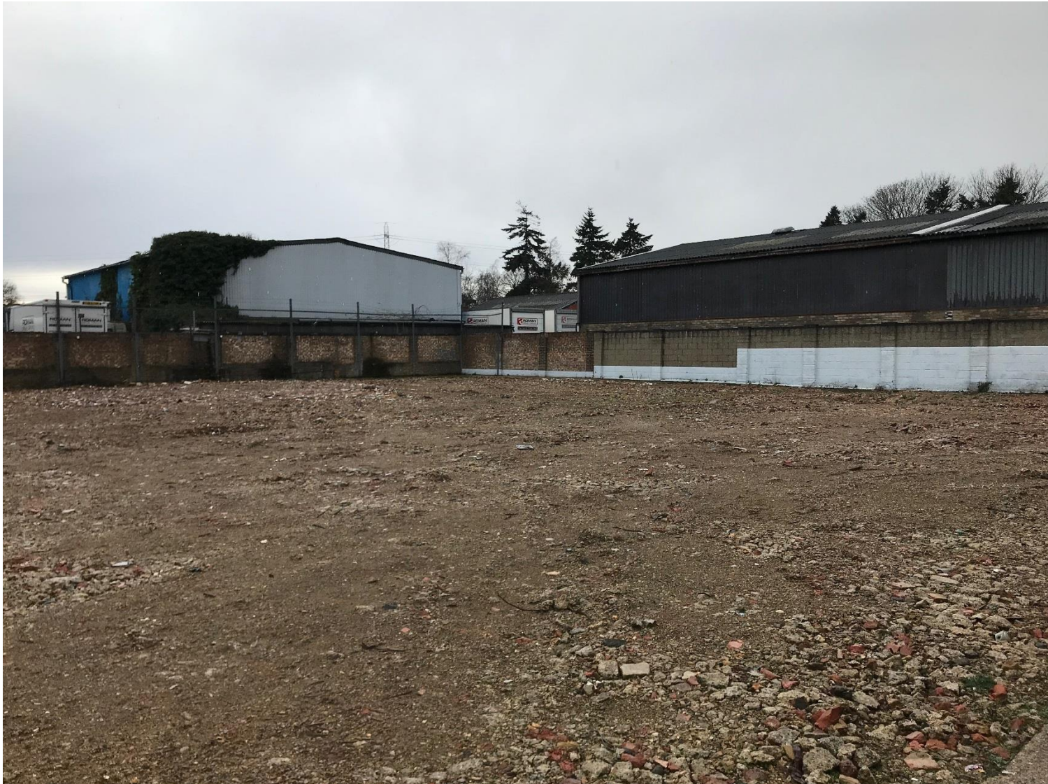
Photo 8: View of existing open area to the rear of Unit 12, looking north-west (location of proposed recycling building).
