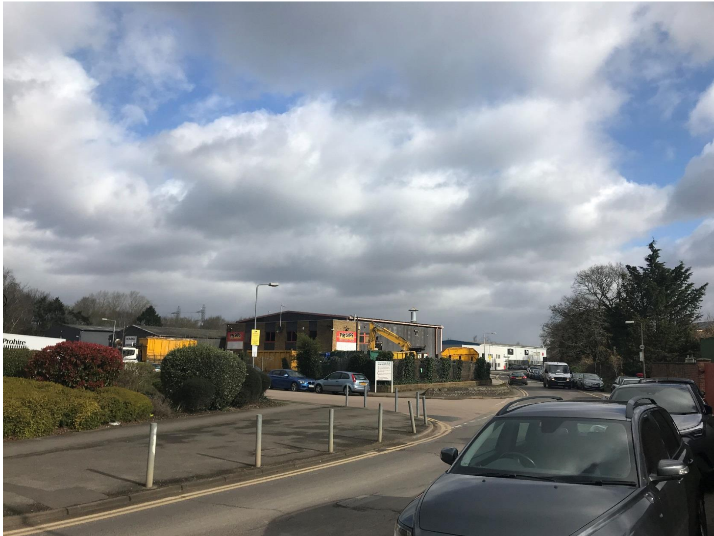
Photo 12: View from Wintersells Road looking north-east towards Unit 10 PM Skips.
